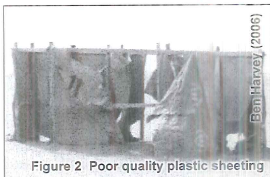
Figure 1 Poor quality plastic sheeting
